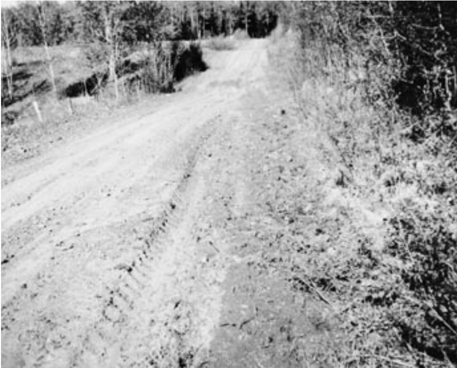
◀ Ruts. No ditch or aggregate.
