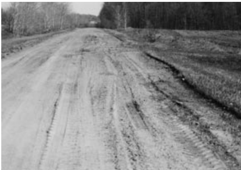
Flat crown with poor grading has created secondary ditch preventing free drainage into roadside ditch. ▼
