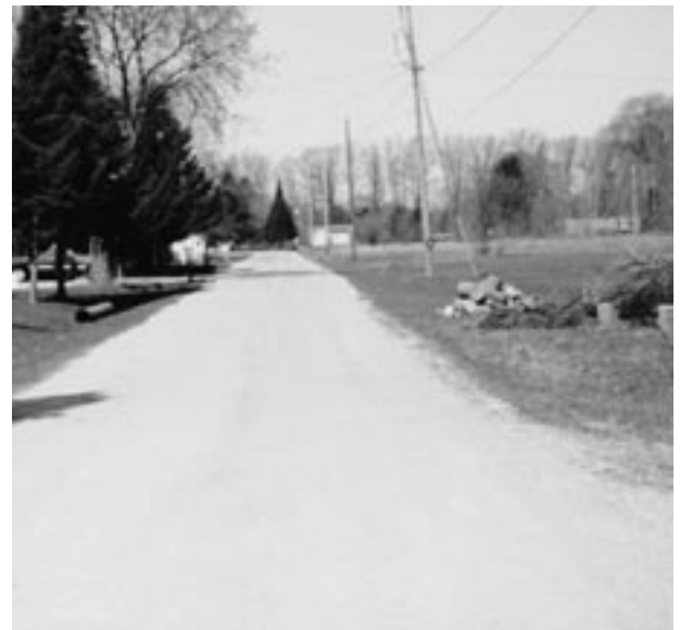
Partial drainage. Ditch and new culvert being added on left. Little or no drainage on right.
