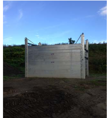
Photo left: Trenching & Shoring held at Johnson Municipal Town Offices and Johnson Town & Johnson Village highway garage.
