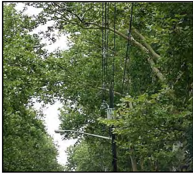
Directional pruning can train the canopy to grow away from or over conductors.
