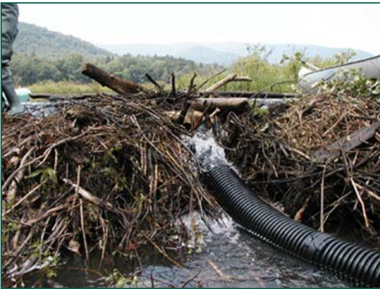
Patching the dam to secure the outflow pipe in place.
