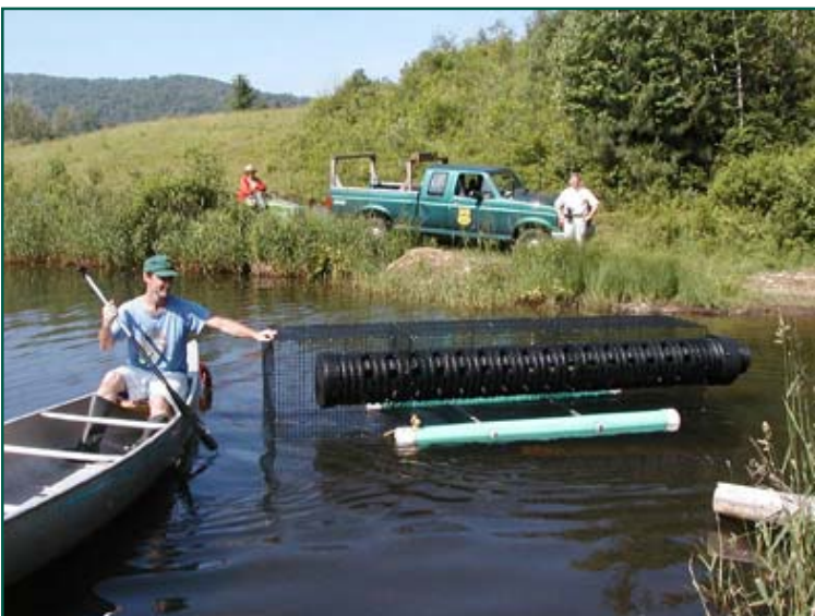
Floating the baffle to the dam.
